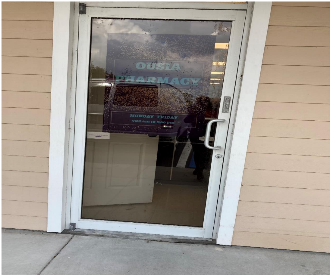
Exhibit 1 Locked Front Door of Pharmacy with no sign for the public to enter from the side.
